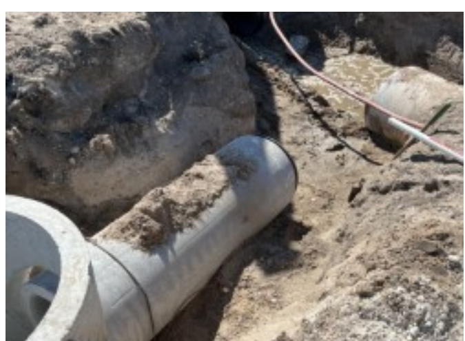
Storm Drainage Construction
