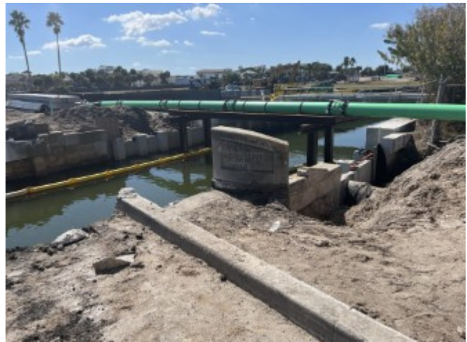
Temporary Support and Forcemain Relocation
