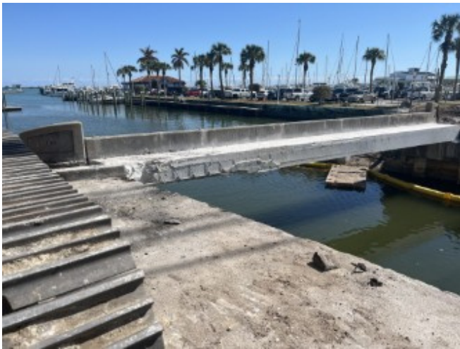
Demolition of the Moore's Creek Bridge
