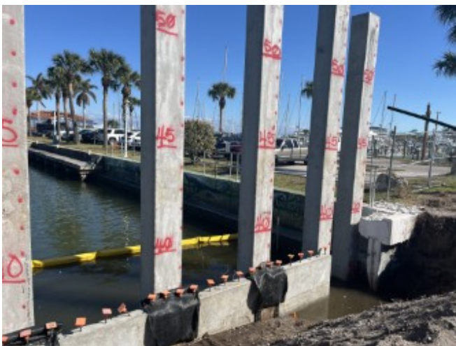
Pilings and Wall Panels
